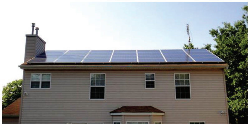
Figure 2: SolarEdge allows for full roof utilization despite shading elements (here: chimney). Full roof utilization can only work if the MPPT range of the module-level device goes low enough to prevent module bypass diodes from being activated.
